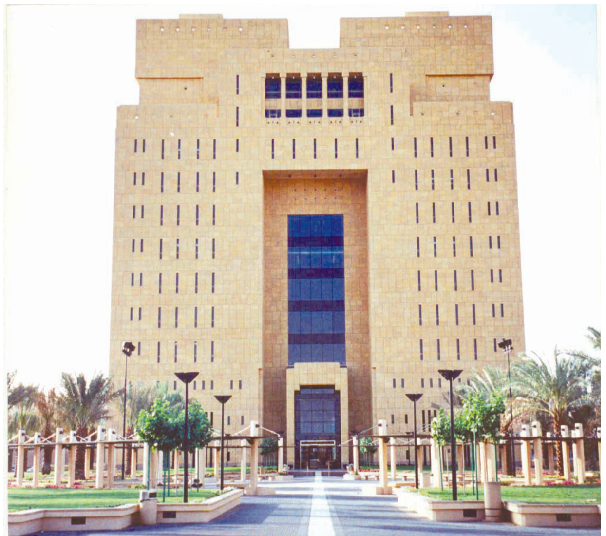
An outside view of the Riyadh Main Court.
